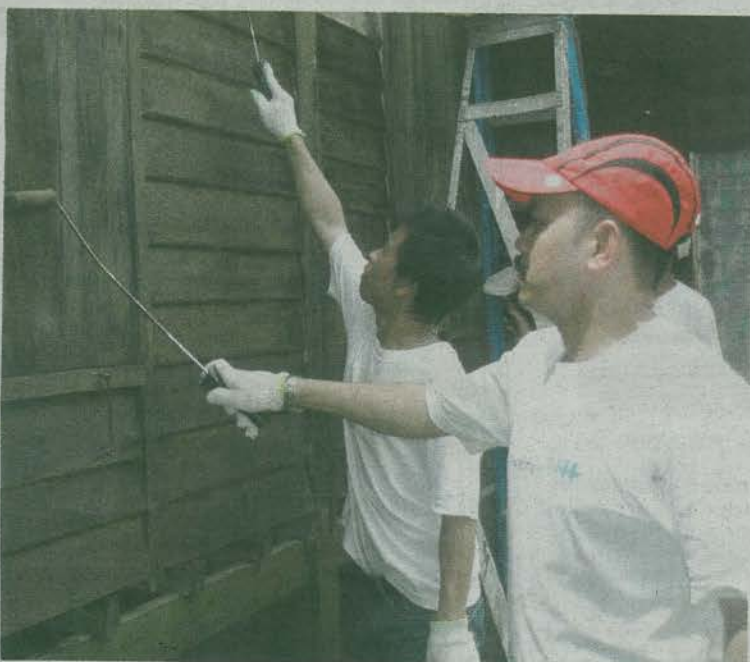
House painting and upgrading in progress
